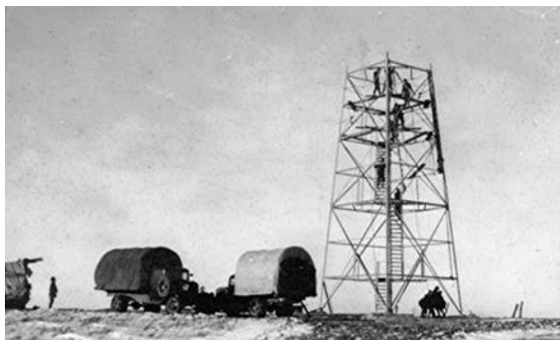
Jersey Hill fire tower under construction by the CCC Crew – March 1935.
